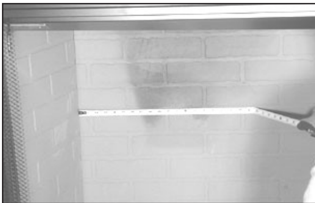
Figure 2.1 Measure Firebox
